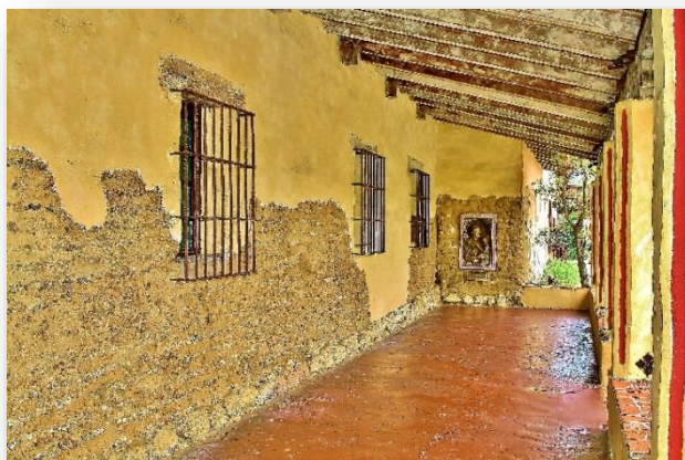
Exterior segment of original adobe wall
