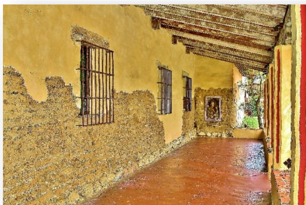
Exterior segment of original adobe wall
