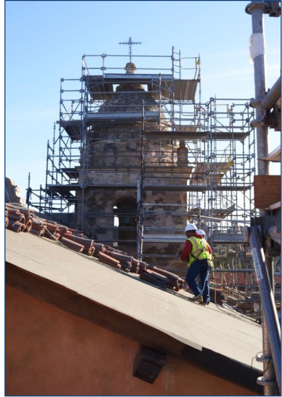
Reinstallation of roof tiles, while dome restoration is underway
