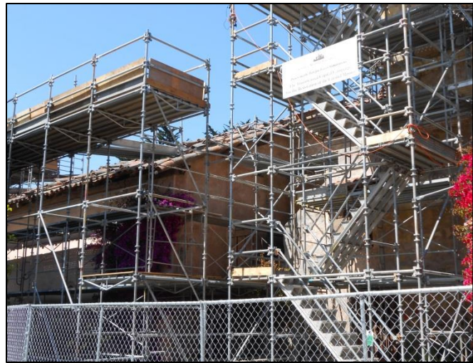
Scaffolding and tile platform on south side of Basilica
