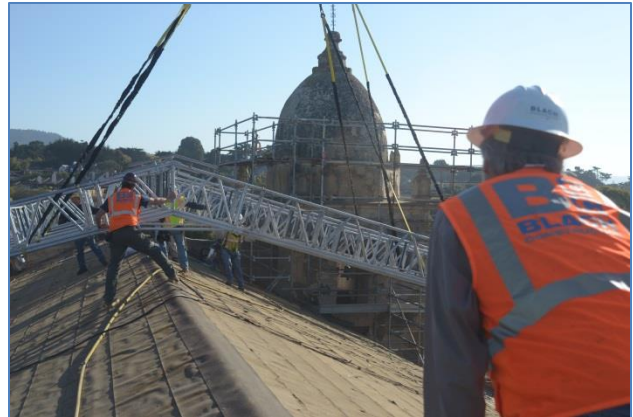
Installing weather protection structure over Basilica
