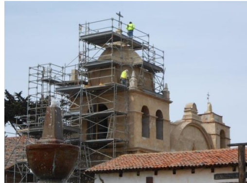
Restoring the bell tower and dome
