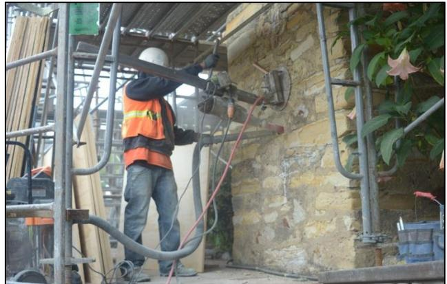
***Core-drilling one of the buttresses***
